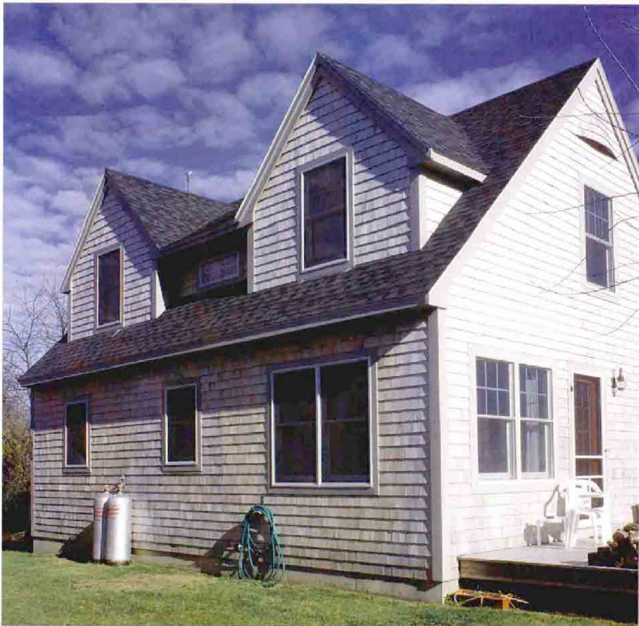
Hybrid dormer. Doghouse dormers create more room and larger egress for the bedrooms at the ends of this house, while the shed room in between creates a space for a full bath. The doghouse-dormer wall is plumbed and braced in place (photo facing page).
